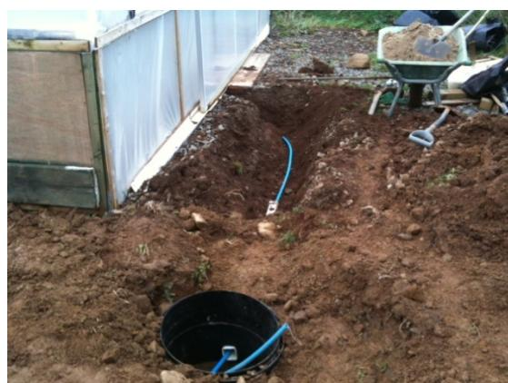
There is a spur ready for our next poly tunnel and a new standpipe, which is on the Southern inside area of the existing poly tunnel
